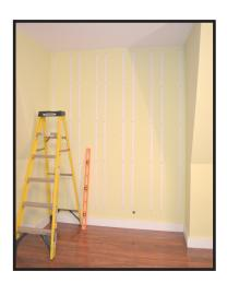
Pressure-fit the panels to the strips, checking for matches along panel edges. Adjust as needed.
