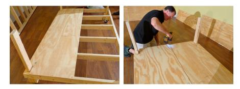
On the inside of each leg, measure down 3 <sup>1</sup>/<sub>2</sub>" and screw in a deck bracket, long leg out. This will hold the weight of the top frame until you get it screwed in.
