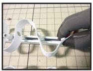
If using a hidden baton, cut the excess tape between the two Master Carrier snaps. Overlap tape so both snaps fit the master snaps. Staple the tape together to hold the spacing.
