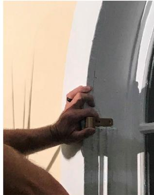
3 Install the top bracket and insert the arched rod into the brackets.
